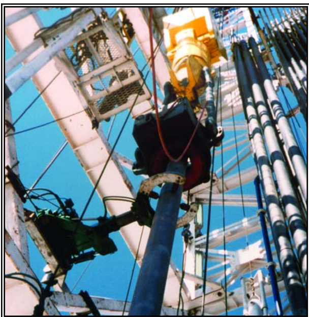
Stab-Rite Guiding Tubular Through 750 ton Elevator
